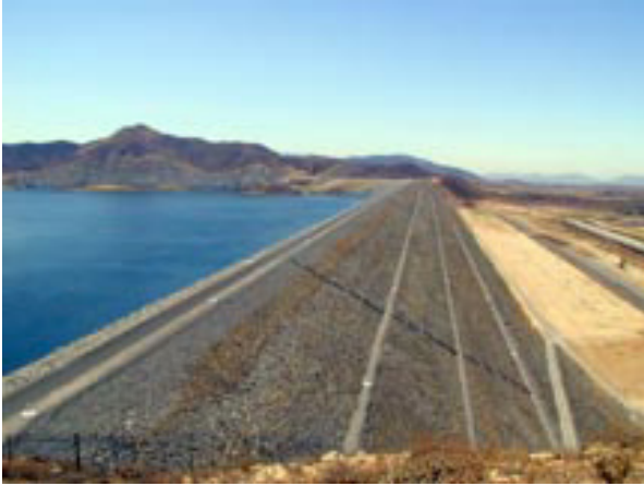
Photo 3: West Dam of Diamond Lake.
